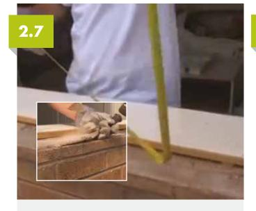
Check that mortar bed has sufficient clearance, if not remove it.
