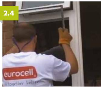
Remove as much glazing as possible, this will help to reduce the weight and allow easier handling.
