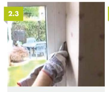
Run a sharp blade around the inside perimeter of the window to break the bond between frame and the plaster. This will also minimise the damage to any interior decoration.
