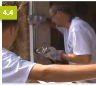
Check that frame is both level and plumb, then drill fixing holes into the frame sides. These should be drilled approximately 150mm from the top and bottom corners and approximately 600mm in between (a minimum of 2 fixings per side)
