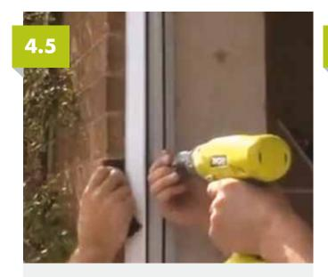
Fix the side of the frame to the wall. Use packers at the fixing points to avoid distortion to the frame and to maintain the 5mm expansion gap. **Do not over tighten the fixings!**
