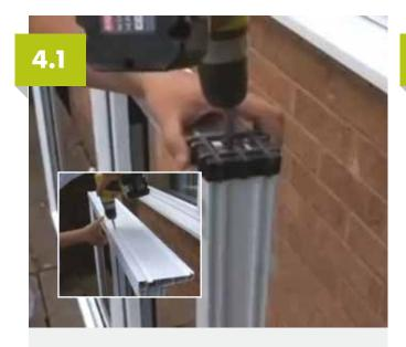
Remove any packaging from the new frame. Apply a bead of silicone along the length of the frame where it will meet the cill. Screw the cill onto the bottom of the frame. Make sure you select a screw that will not penetrate the inner skin of the frame.
