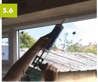
Run a strip of masking tape around the frame, then apply a bead of sealant between the frame and the wall. Remove the tape before the sealant sets. Apply this step to all four sides of the frame.
