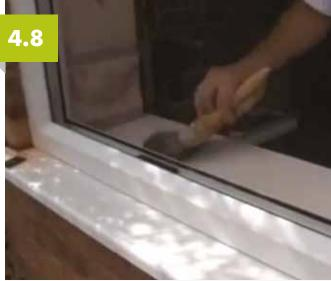
Before reaching the final stages, clean any brick dust or debris from the frame and surrounding areas.
