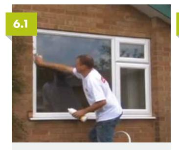
Clean the external surfaces to remove the dirt and grit.
