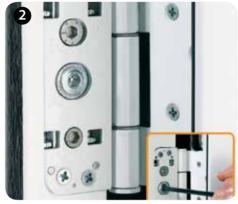
Use a 5mm Allen Key for independent compression, horizontal and lateral adjustments.
